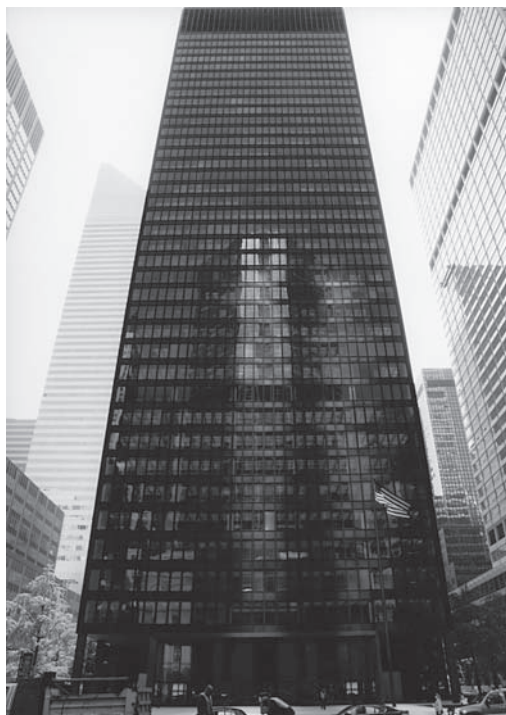
Figure 6. Mies van der Rohe and Philip Johnson, Seagram Building, New York City, 1954–58. (Image in the public domain.)
