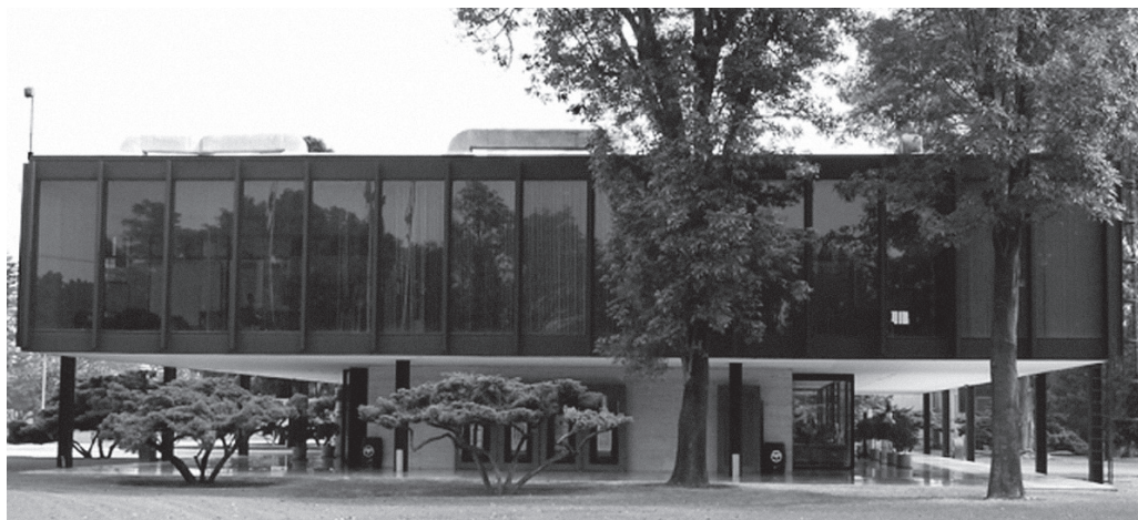
Figure 8. Bacardi Administration Building, side view. (Photograph by author.)
